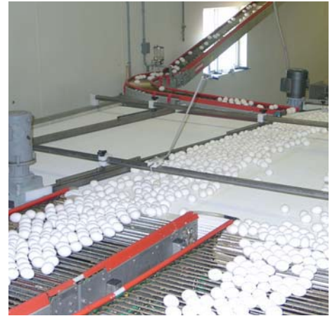
Installation of Curve Conveyor, Transfer Table and Dirty Egg Return Conveyor
